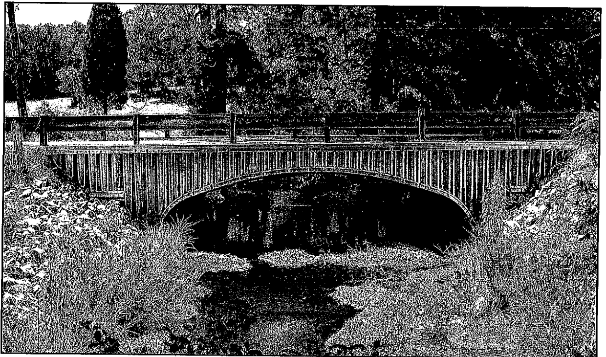
Aluminum Box Culvert - stream crossing
