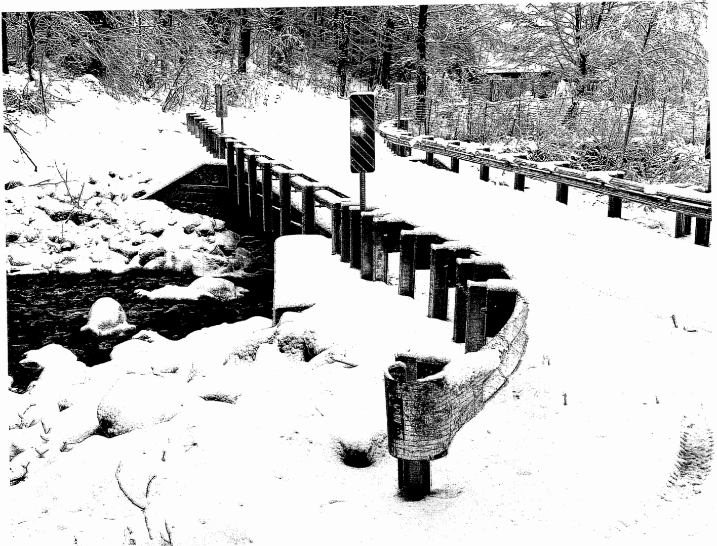
New bridge on Churchill Road Photo by David Atherton
