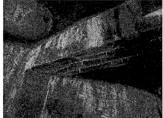
Cracking and Efflorescence in the Bottom of Beam 3
