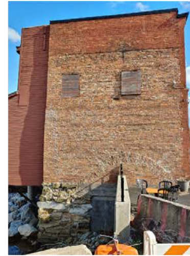
Historic North Facade of Blue Moon Building (Mortar repair w/possible mural project)
