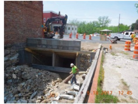
^ Culvert construction phase - 2017
