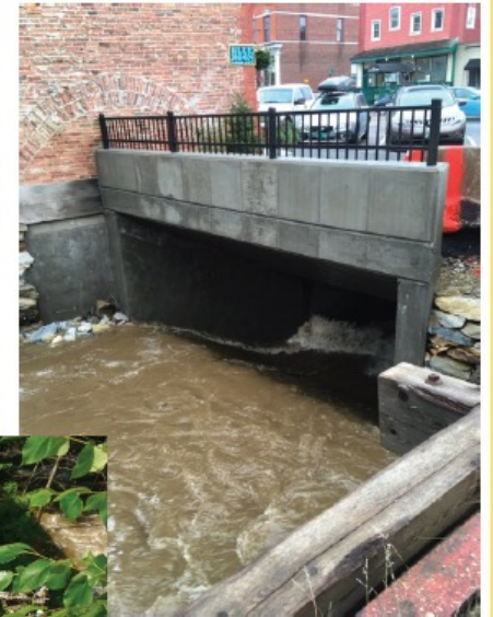
Culvert at work in 2018 storm ^
